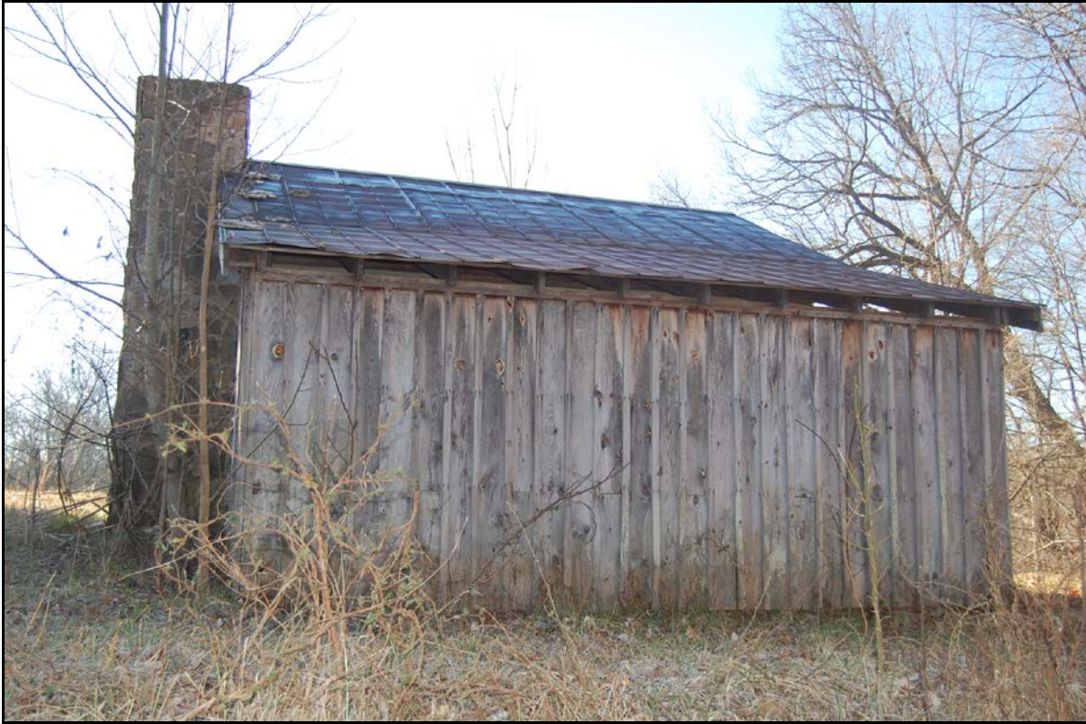
Figure 12. Dellinger Road Log House: north rear and east side elevations
