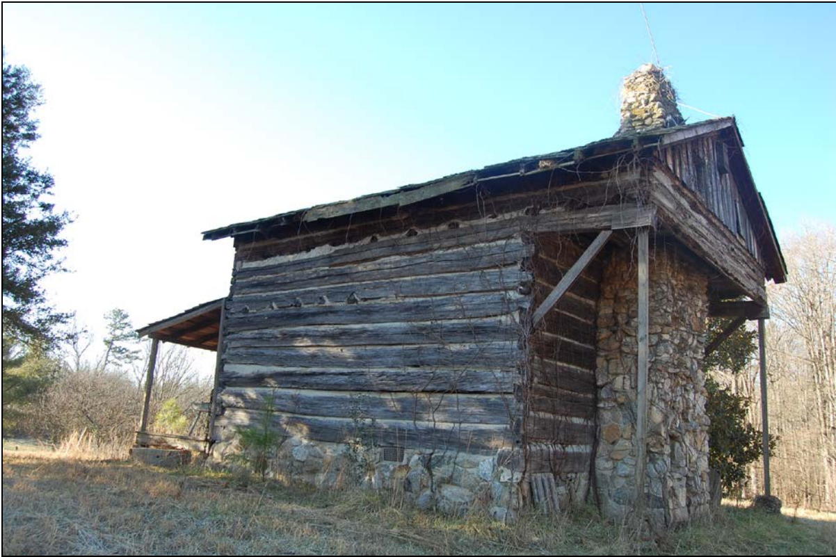
Figure 8. Glasco Cabin: east side and north rear elevations
