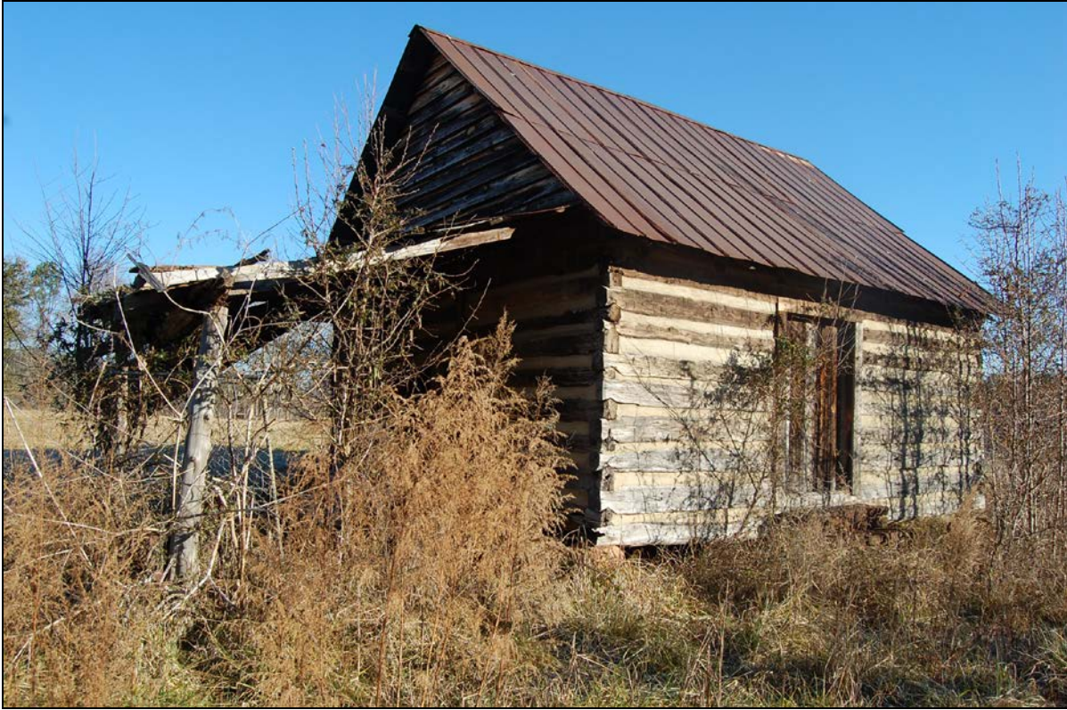
Figure 14. Dellinger Road Log Barn: south and west gable-end elevations
