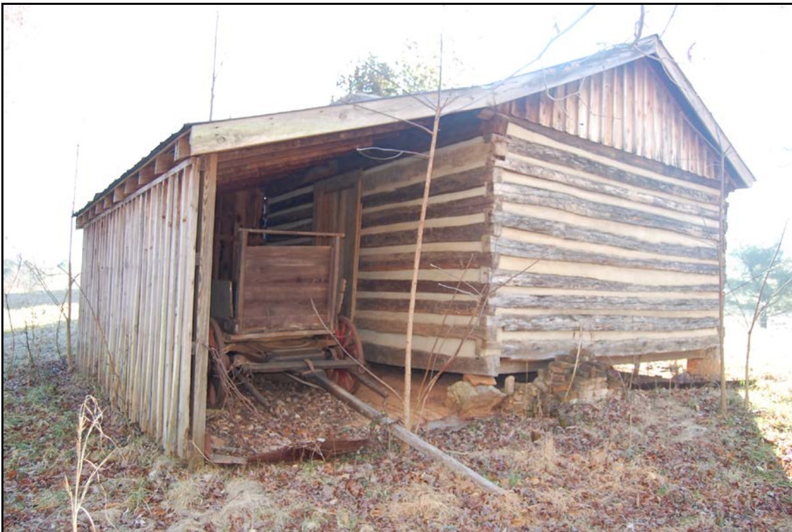
Figure 11. Dellinger Road Log House: west side and north rear elevations
