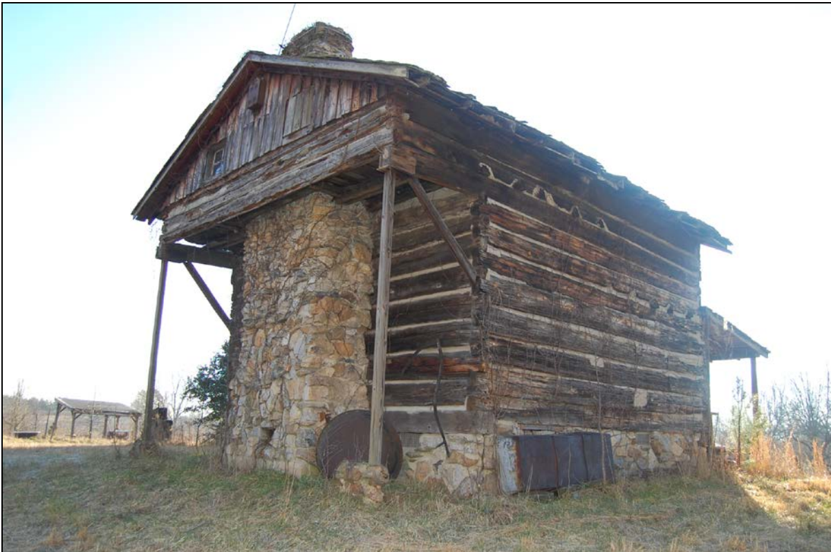
Figure 7. Glasco Cabin: north rear and west side elevations
