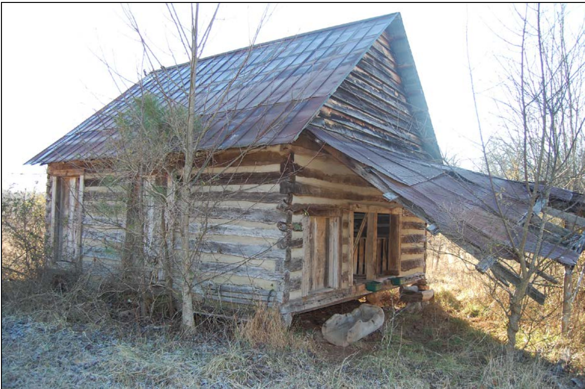
Figure 15. Dellinger Road Log Barn: west gable-end and north elevations
